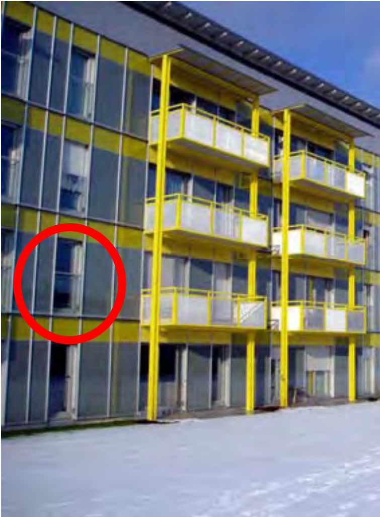
Fixed glazed window parapet
